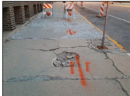
Earlier this year, Connect Transit set up a bus stop along the sidewalk. Complaints soon followed. An inspection by the Engineering Division revealed that the sidewalk, already in poor condition, had rapidly deteriorated in the past year. Public Works closed the sidewalk and the bus stop had to be relocated. Temporary patching options were examined but staff concluded that the damage is too extensive to make patching practical.
